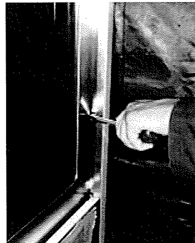
Figure 3-24. Pry into Door Frame
