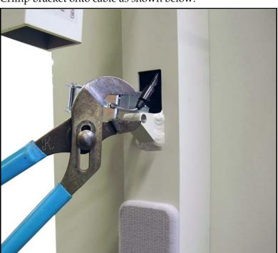
**12** Crimp bracket onto cable as shown below.
